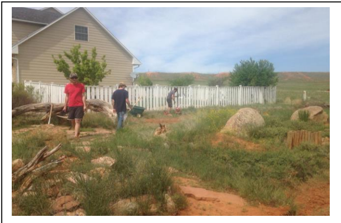
Above: Installing trenches and landscaping. By Jane Greaser
